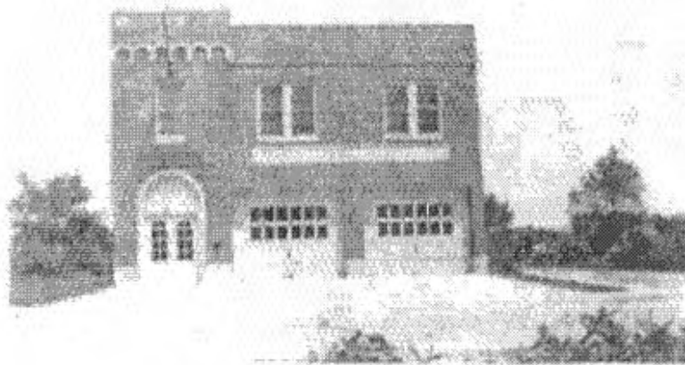
Frankford Fire Hall (before Addition) Main Street
